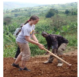
Anastacia helping clear the loose dirt.
